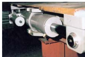
Pot Bearing with Shock Transmission Unit MSTU
